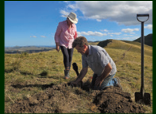
Jen and Chris installing a new water line.
